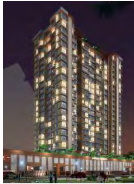
ANSHUL HEIGHTS - A & B Wing Kandivali (West) Completed in 2019
